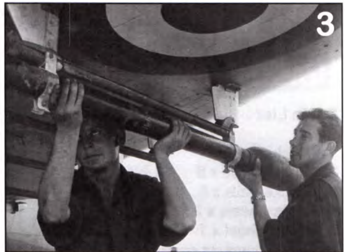
Armourers fitting a rocket to the launch rail. Note the clamps holding the rocket which allowed a second tier to be fitted.
